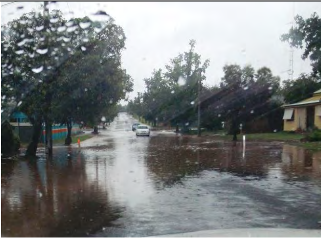
Plate B1.1 – 7/03/2010 16:29 hours - Looking north along Charles Street south of Kiesling Lane (Source: Council)
