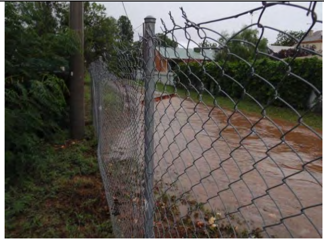
Plate B1.8 – 7/03/2010 16:39 hours - Looking north along open drain, silt basin (Source: Council)
