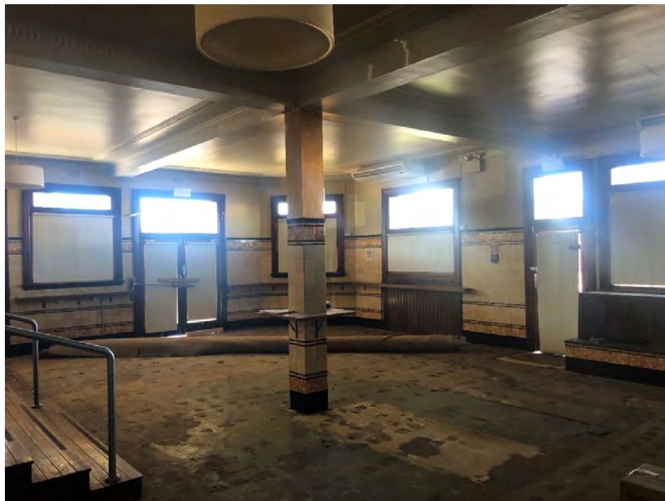
Internal looking to the front
