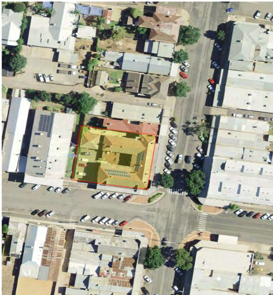
Development surrounding 100-106 East Street Narrandera (Source: LPI Six Maps)
