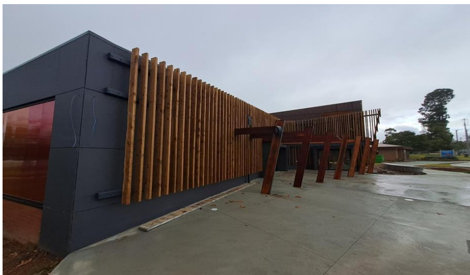
Front (Eastern) view under construction– Destination & Discovery Hub
