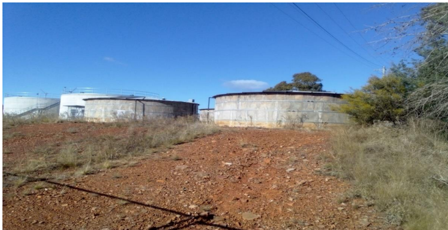
Redundant water tanks – Pine Hill
