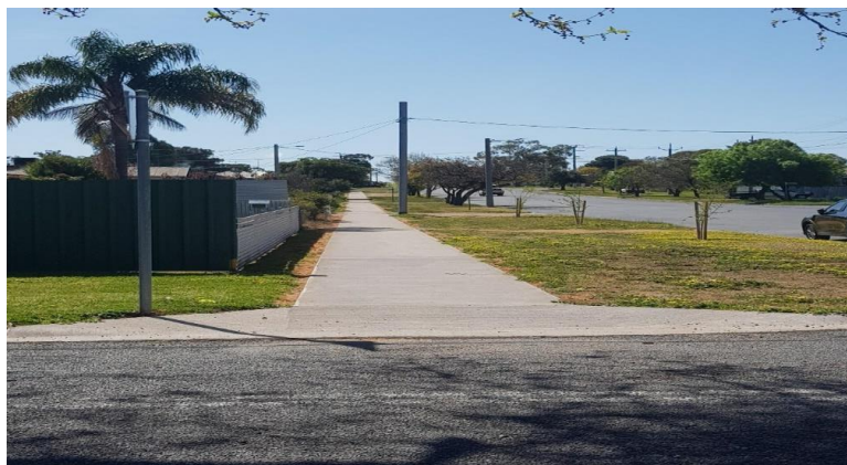
Completion of the Adams St section of the footpath
