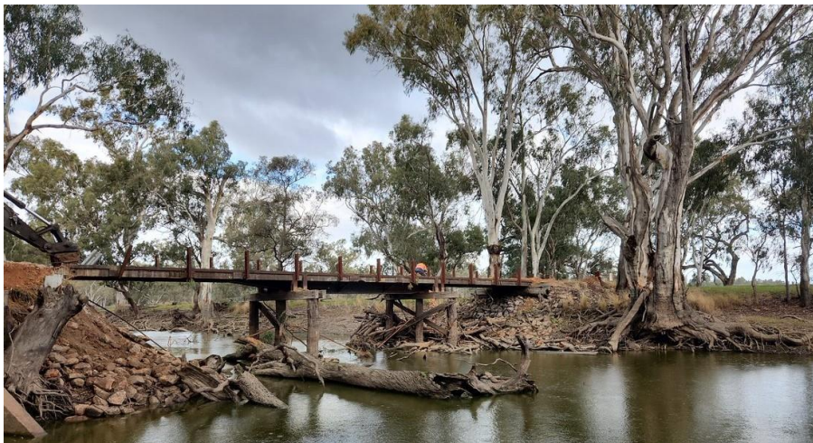
Mollys Bridge during works
