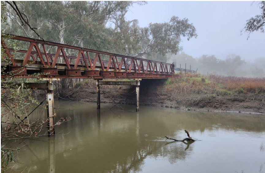
Somerset Bridge before works
