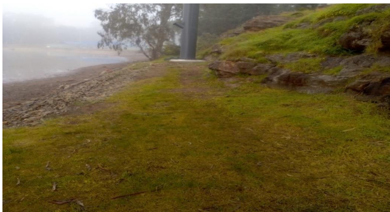
Site of pedestrian deck – Lake Talbot Water Park– Under construction.
