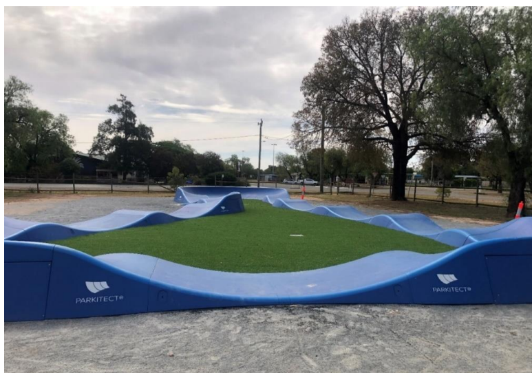
Pump track installed at Barellan Sportsground
