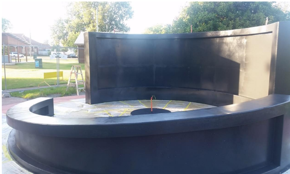
The Wiradjuri wall – Under construction – Looking south – Marie Bashir Park
