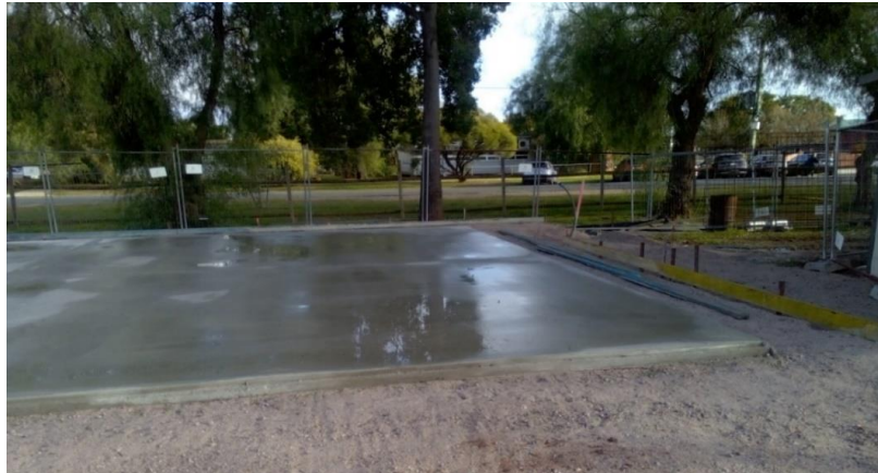
Concrete floor - new spectators pavilion – Barellan Sportsground
