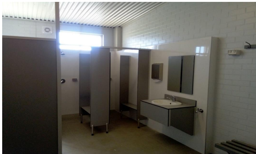
Refurbished umpires changerroom – Narrandera Sportsground
