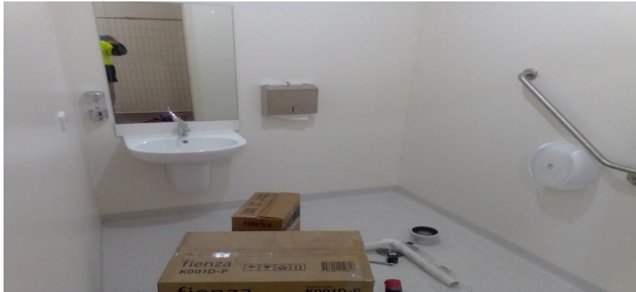
New accessible unisex toilet – Under construction – Narrandera Tennis Club
