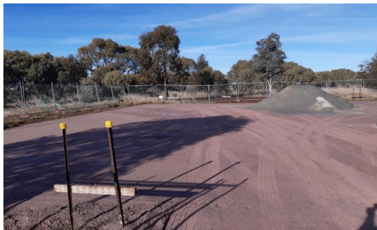
Earthworks underway – Landervale Fire shed
