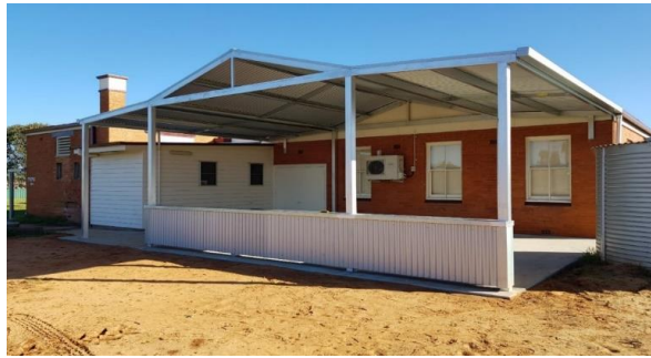
The new covered pergola at the rear of the Hall
