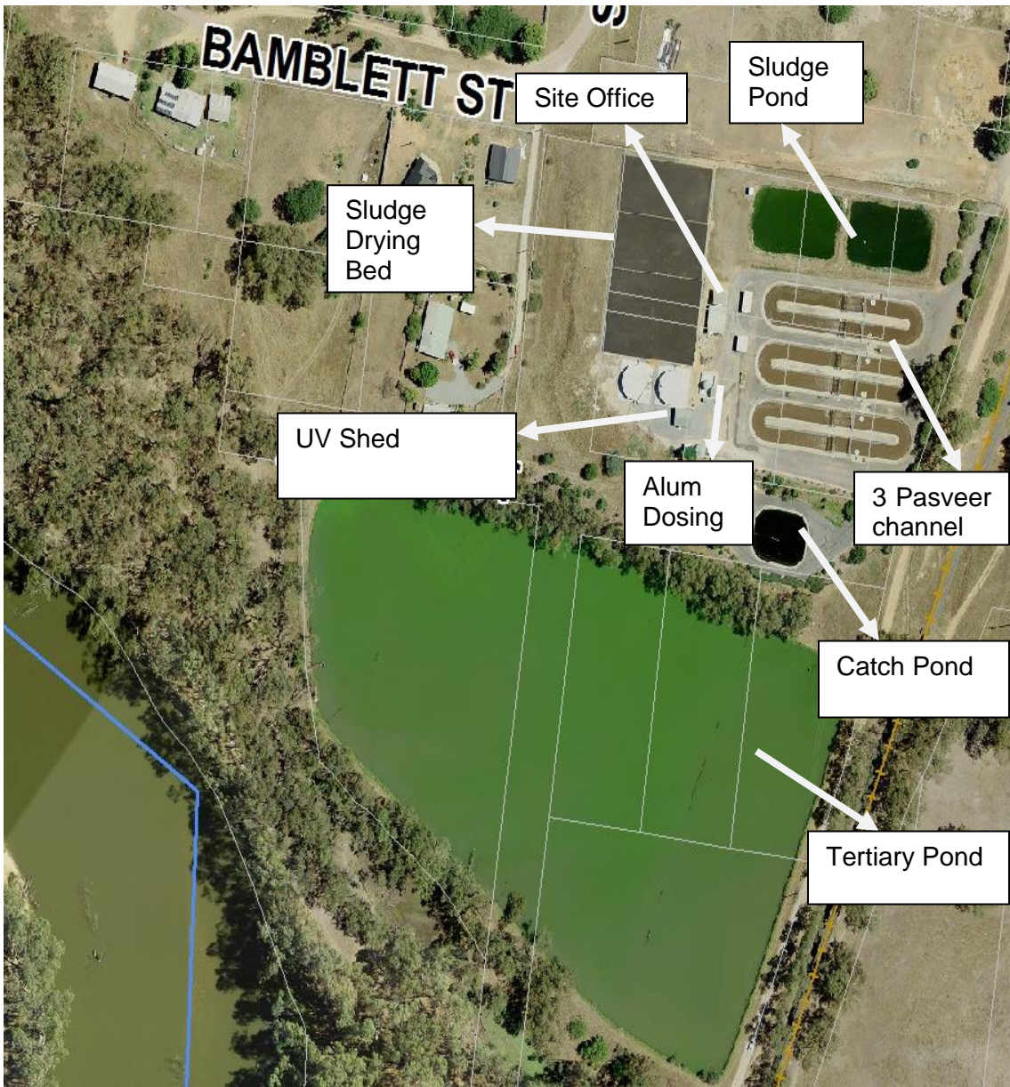
Narrandera Sewer Treatment Plant
