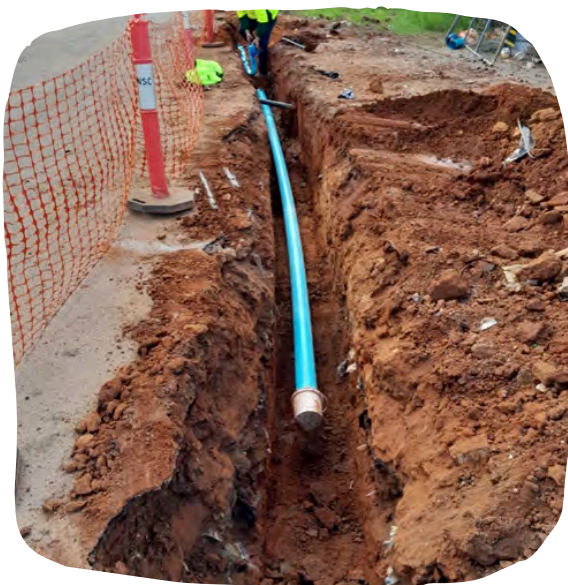
Narrandera landfill water main extension
