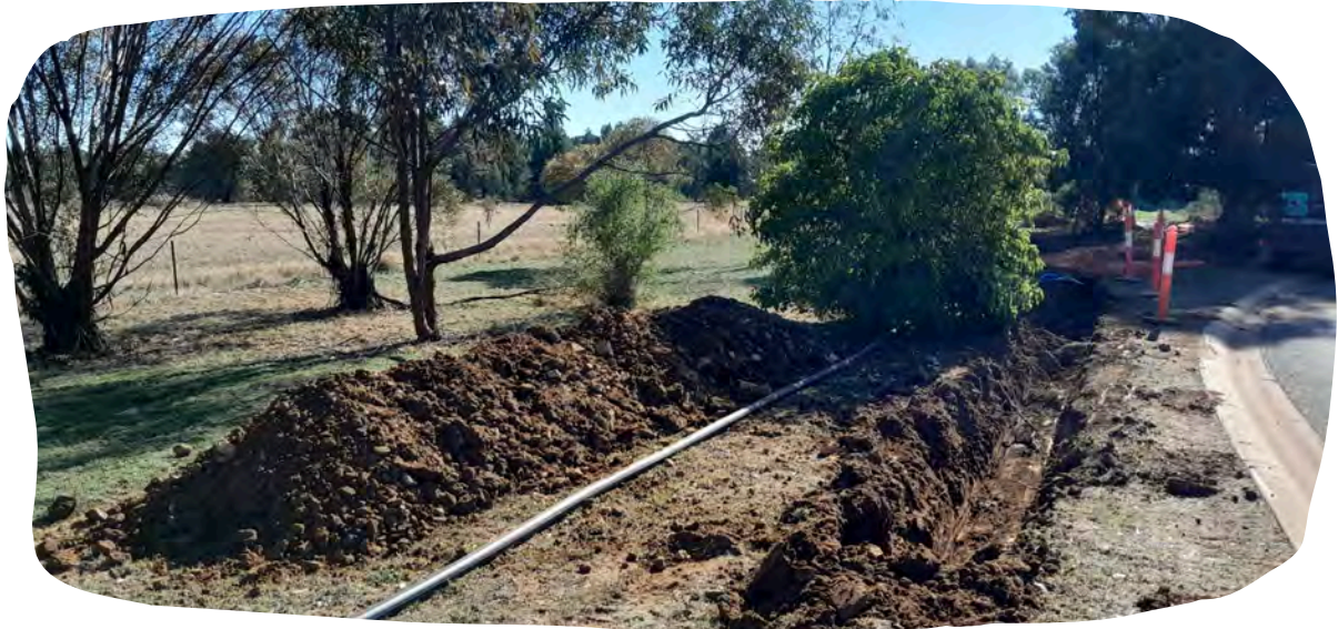
Water main extension in Anzac Crescent
