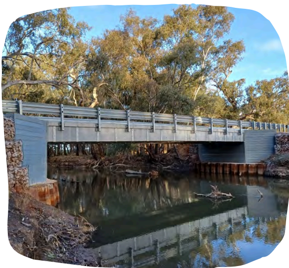
Somerset Park Bridge (Back Yamma Road)
