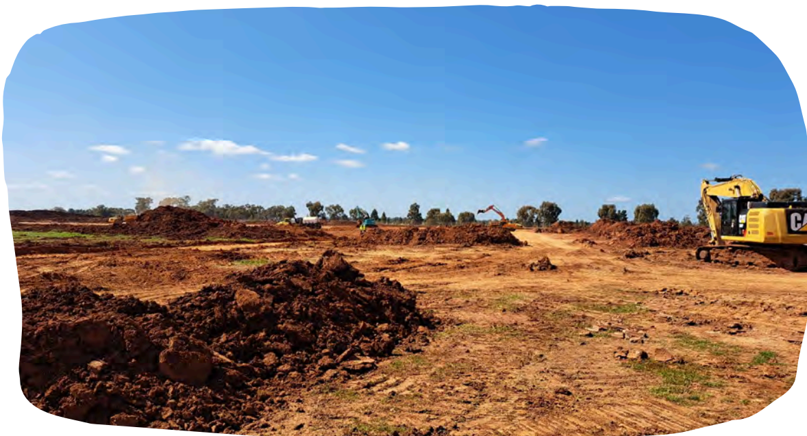
Construction of Sewer Treatment Plant adjacent to Kolkilbertoo Road
