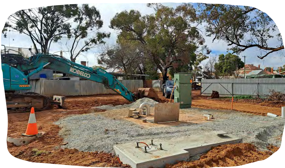
Construction of a Sewer Pump Station at Barellan
